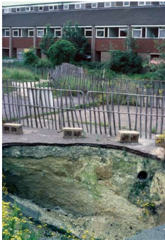
Figure 4.4 One of the collapses in Jacqueline Close, Bury St Edmunds, with the abandoned houses behind. The profile in the collapse reveals the tarmac on 30 cm of roadbase, with a broken drain on the right, on almost structureless putty chalk.
